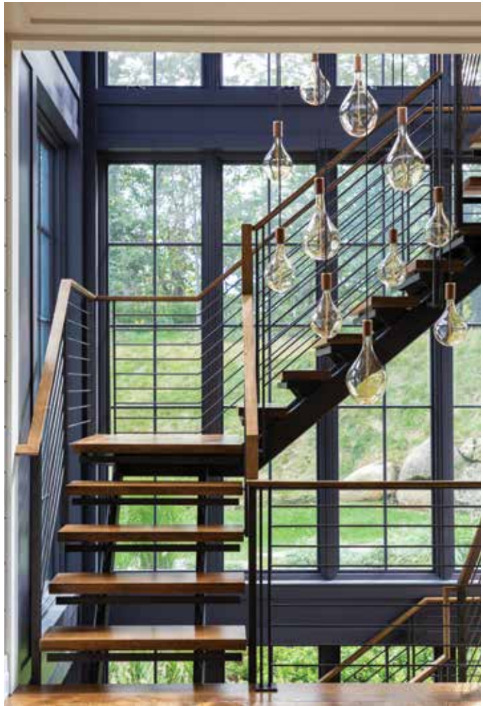
ABOVE: Operable windows in the stair bays let cool air come in around the gardens and hot air dissipate out the top. LEFT: Large bifold doors unite the family room and covered porch, creating an immersive indoor-outdoor experience.
